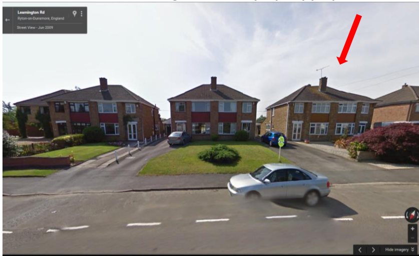
Photo1 – View from Leamington Road to property proposed for demolition to provide site access
