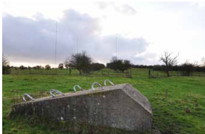
Mast concrete anchors + cables
