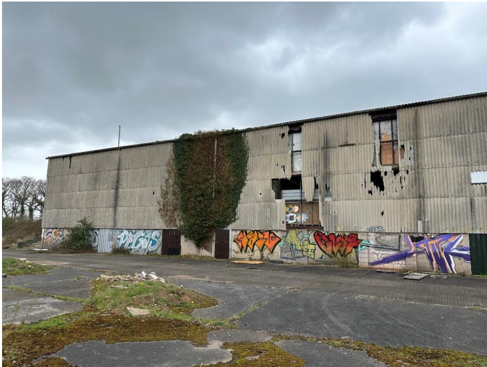
Plate 43 Main Grandstand western rear elevation
