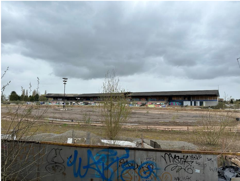
Plate 3 View West onto Main Grandstand
