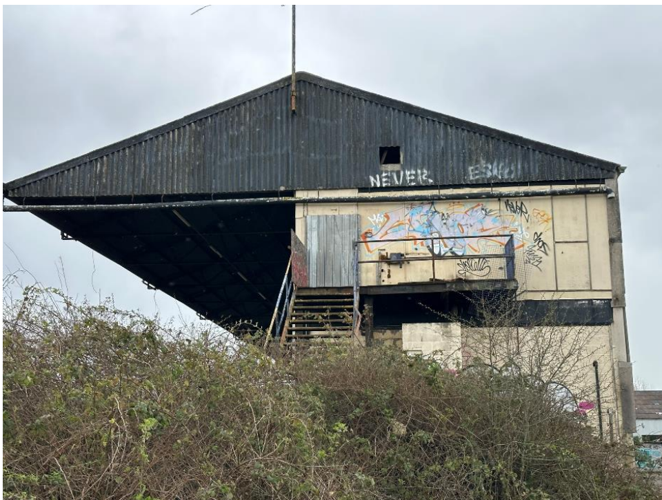
Plate 52 Main Grandstand northern end elevation
