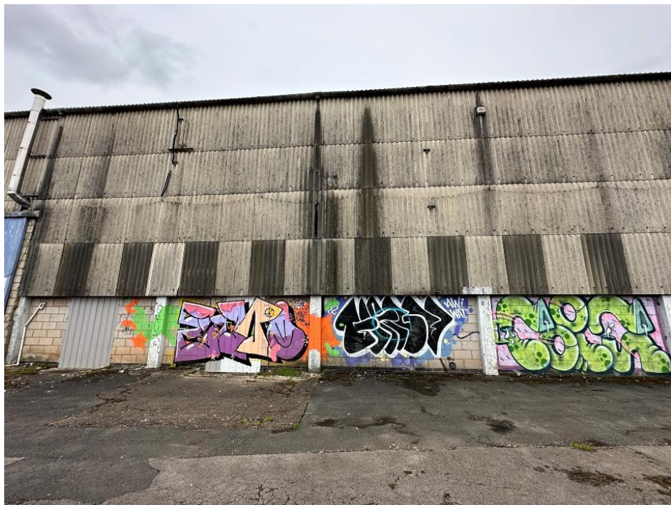
Plate 42 Main Grandstand western rear elevation
