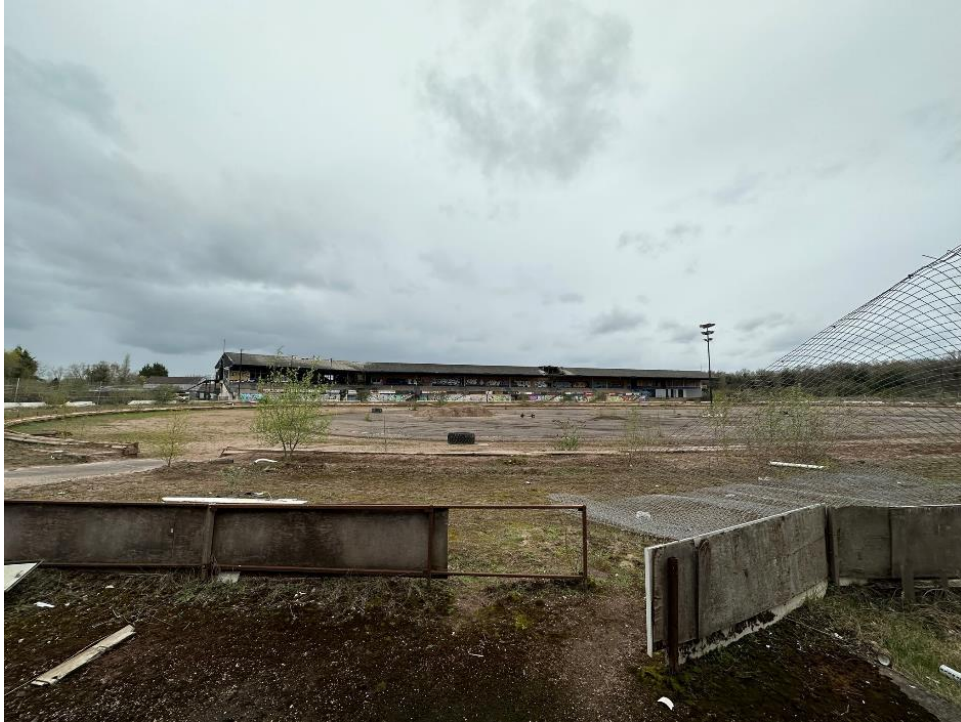
Plate 1 View West onto Main Grandstand
