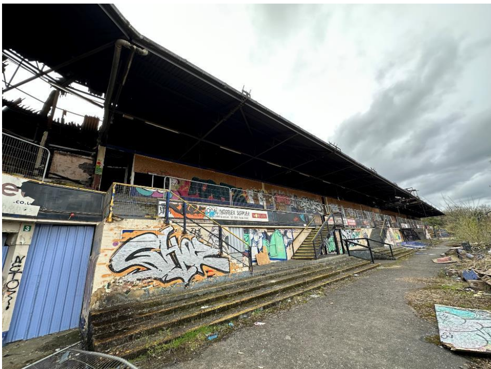
Plate 8 Main Grandstand northern section
