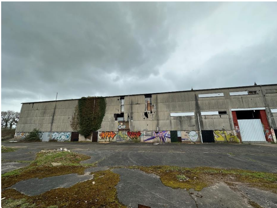
Plate 46 Main Grandstand western rear elevation
