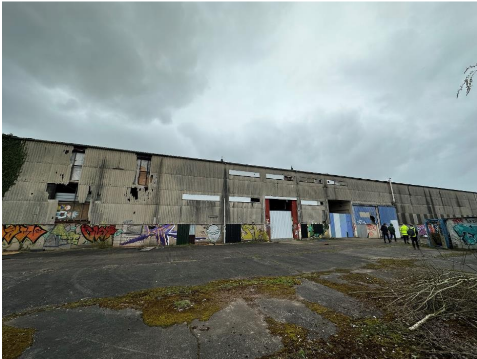
Plate 47 Main Grandstand western rear elevation
