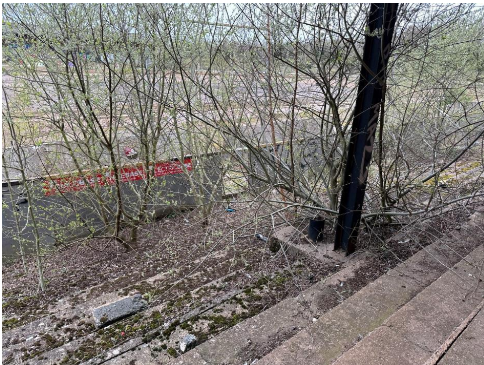
Plate 66 Eastern Grandstand terrace self seeding planting growth unseating
