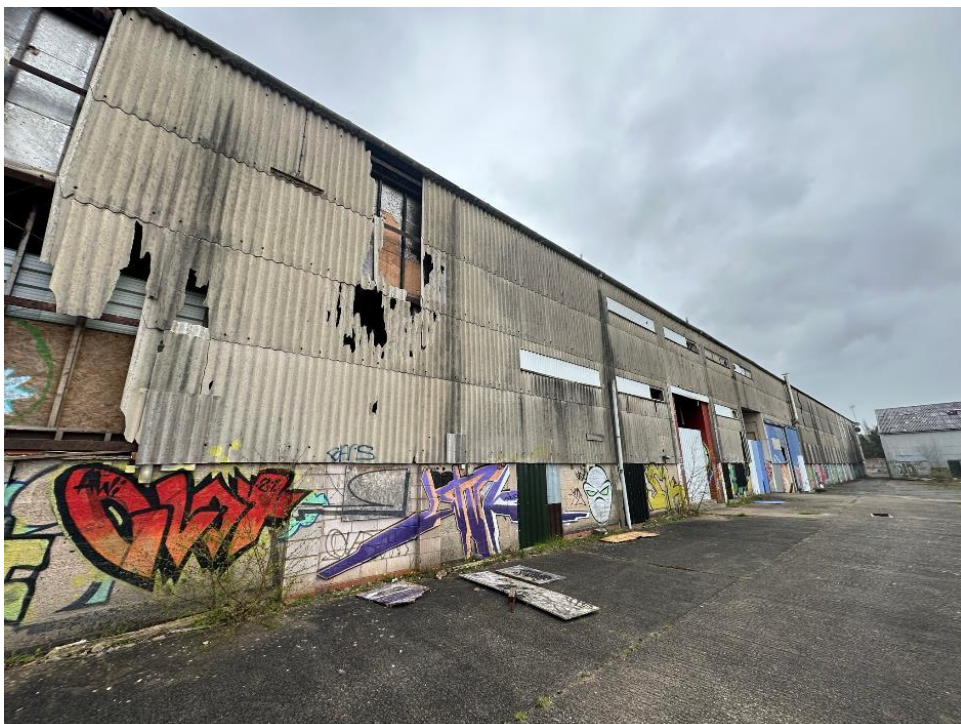
Plate 48 Main Grandstand western rear elevation
