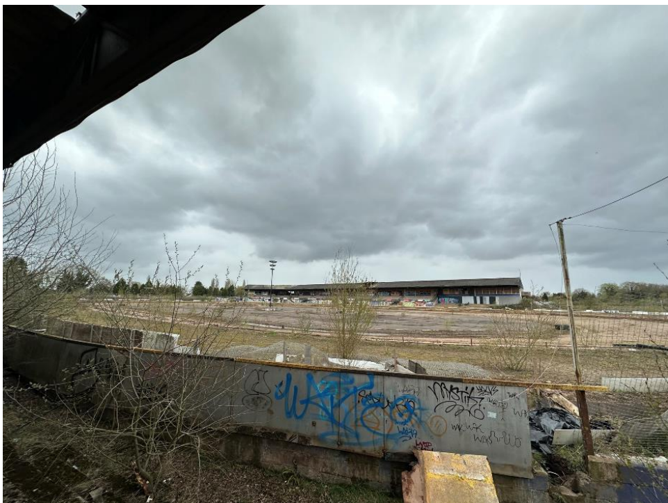
Plate 4 View West onto Main Grandstand
