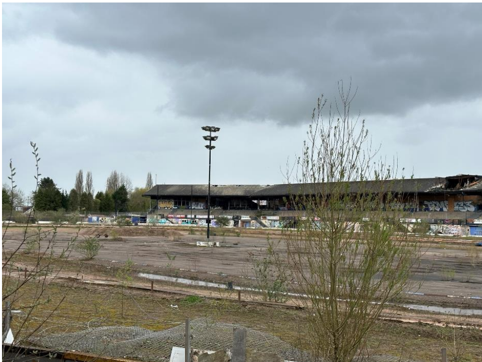
Plate 6 View West onto Main Grandstand
