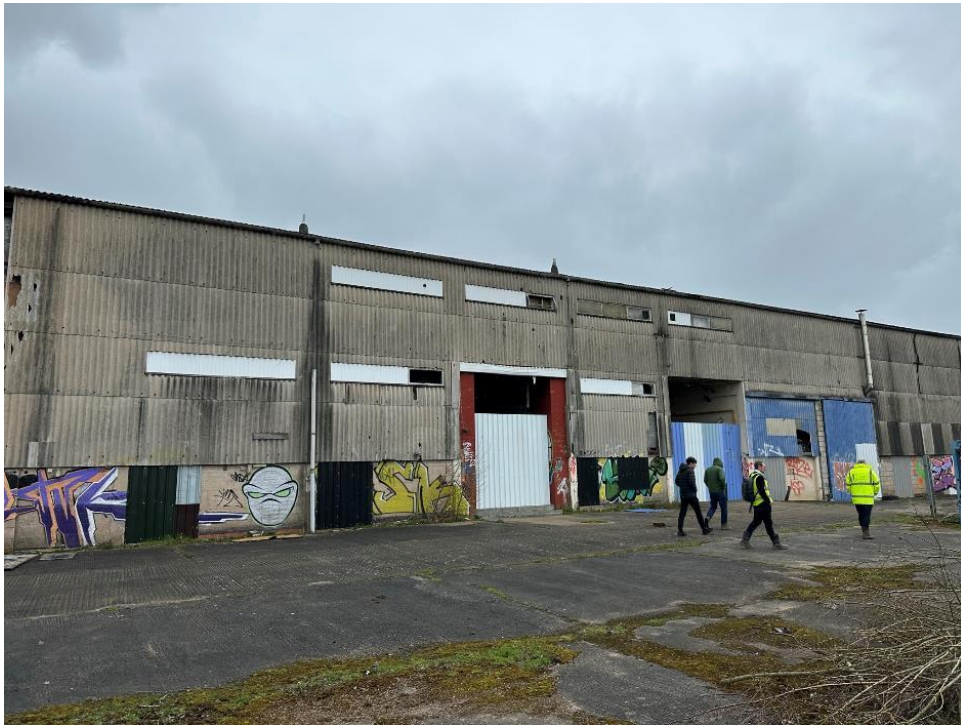
Plate 45 Main Grandstand western rear elevation
