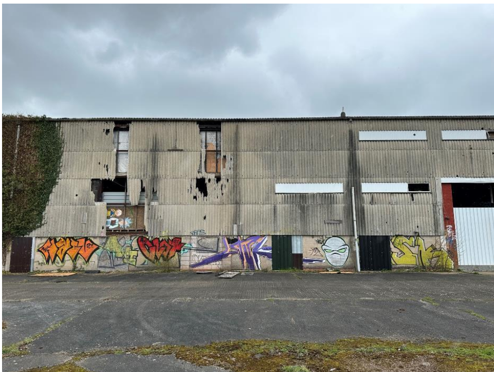
Plate 44 Main Grandstand western rear elevation
