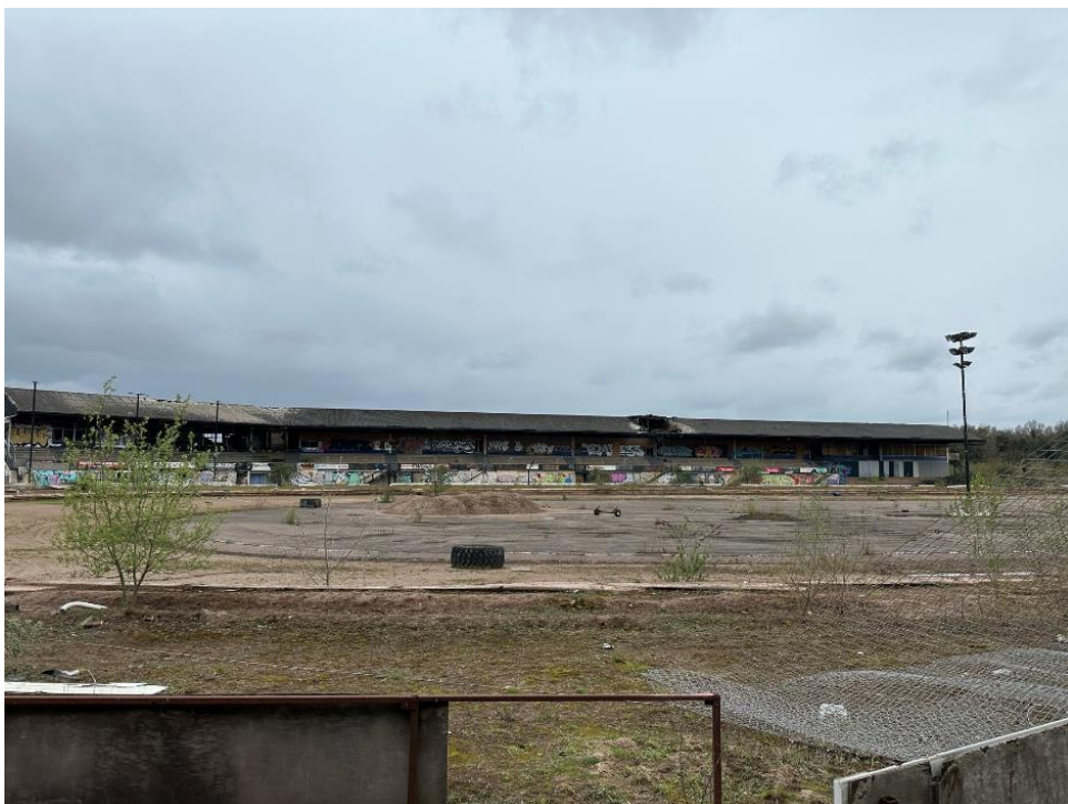
Plate 2 View West onto Main Grandstand
