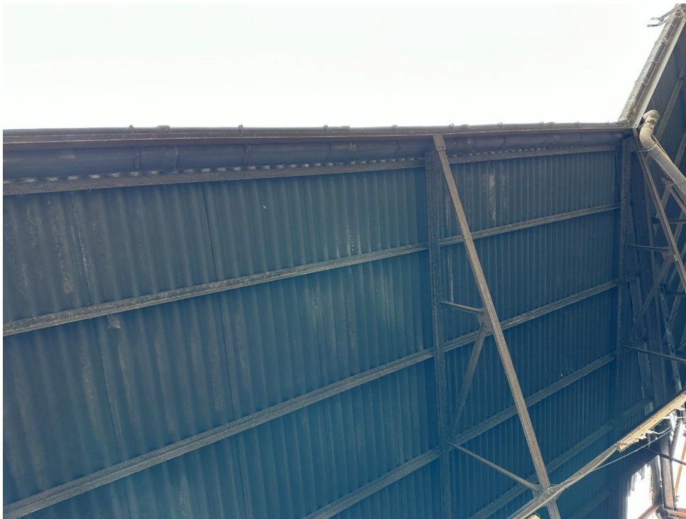
Plate 18 Main Grandstand Roof Structure
