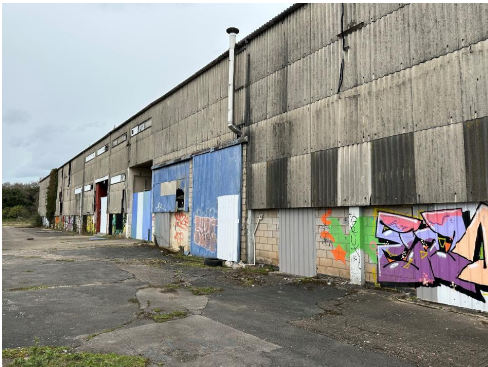
Plate 40 Main Grandstand western rear elevation
