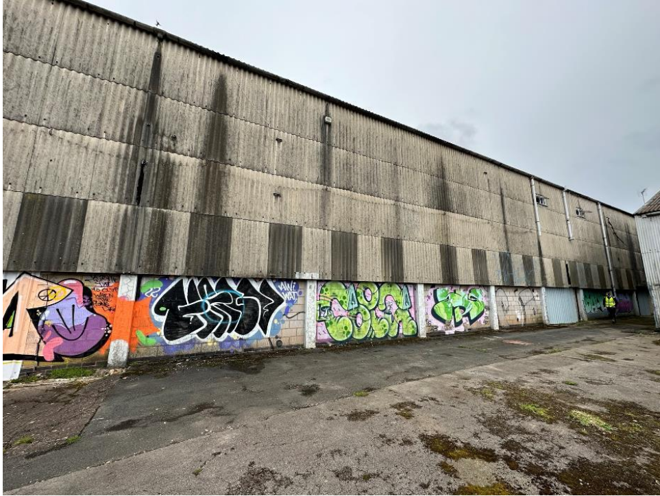
Plate 41 Main Grandstand western rear elevation
