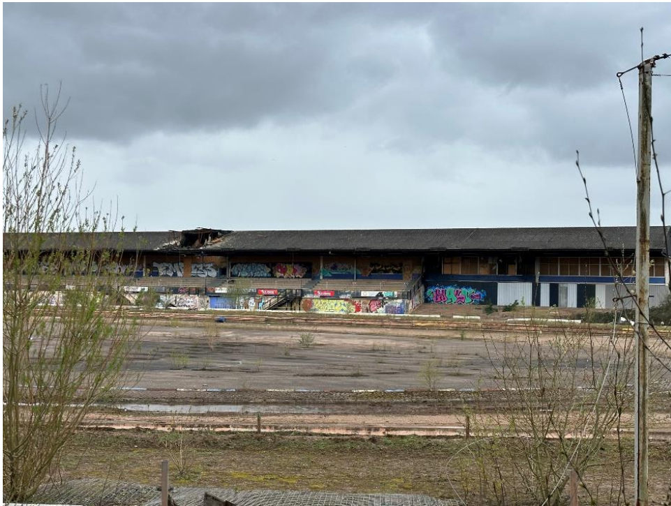
Plate 5 View West onto Main Grandstand
