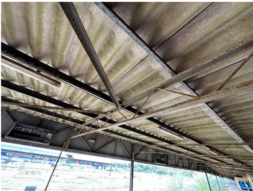
Plate 60 Eastern Grandstand roof structure southern end
