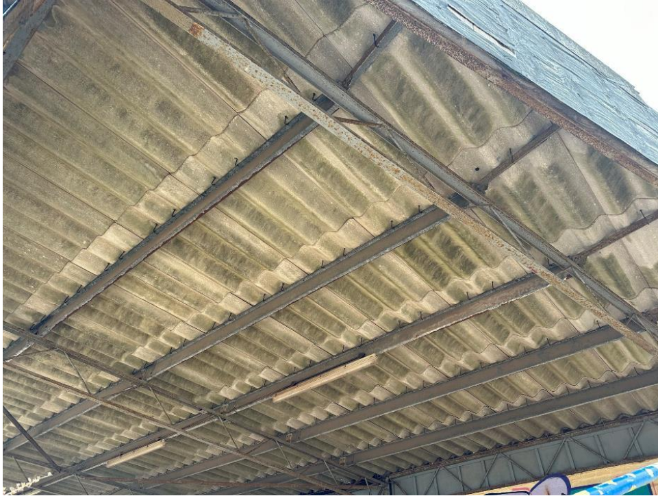
Plate 55 Eastern Grandstand roof structure
