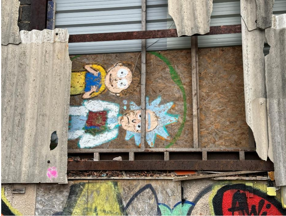
Plate 49 Main Grandstand western rear elevation
