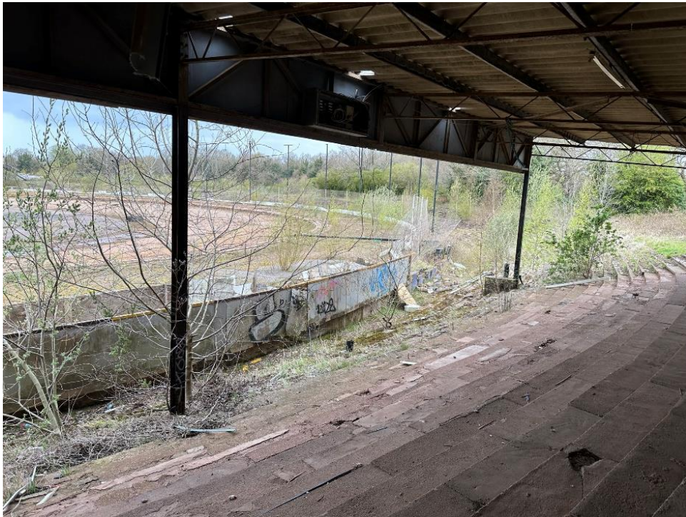
Plate 71 Eastern Grandstand terrace self seeding planting growth unseating
