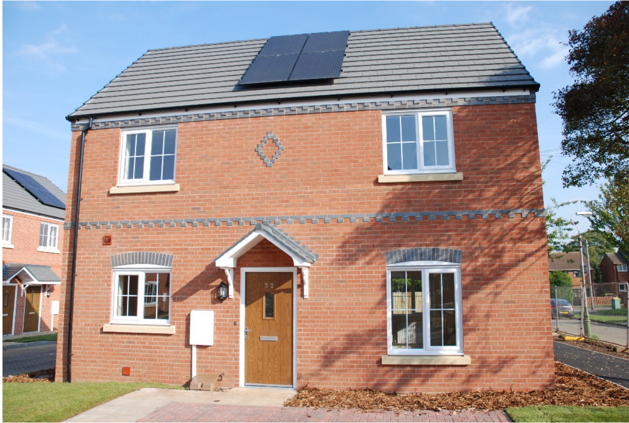
Completed new homes at Pettiver crescent, Hillmorton
