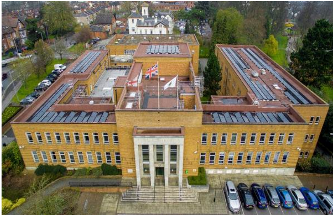
Rugby Town Hall Completed Solar Panel Project
