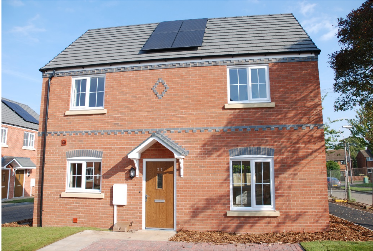
Completed new homes at Pettiver crescent, Hillmorton
