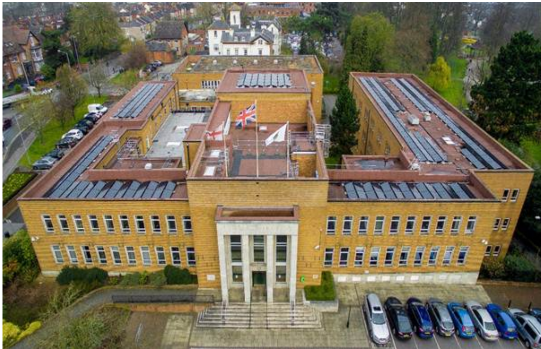
Rugby Town Hall Completed Solar Panel Project
