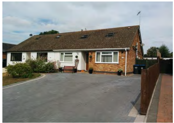
1960s bungalows at the top of Main Street to the right of The Smithy
