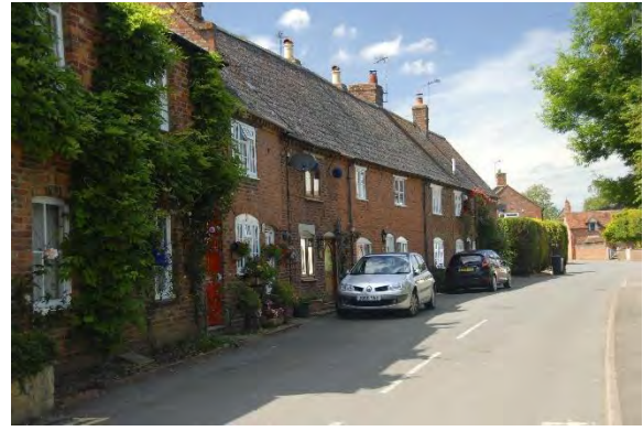
Lower Street Cottages looking north
