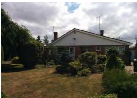
Bungalow with closed gable end facing the road
