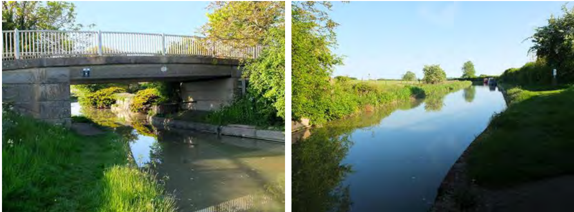
Oxford Canal bridge by Navigation Cottage and View towards Braunston
